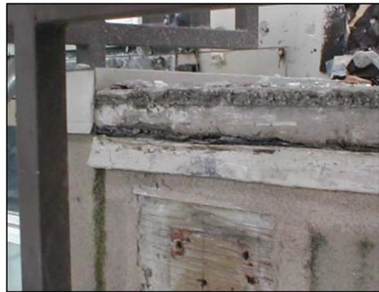
*Balcony Damage Where Flashing and Railings Were Removed After Inspection*
